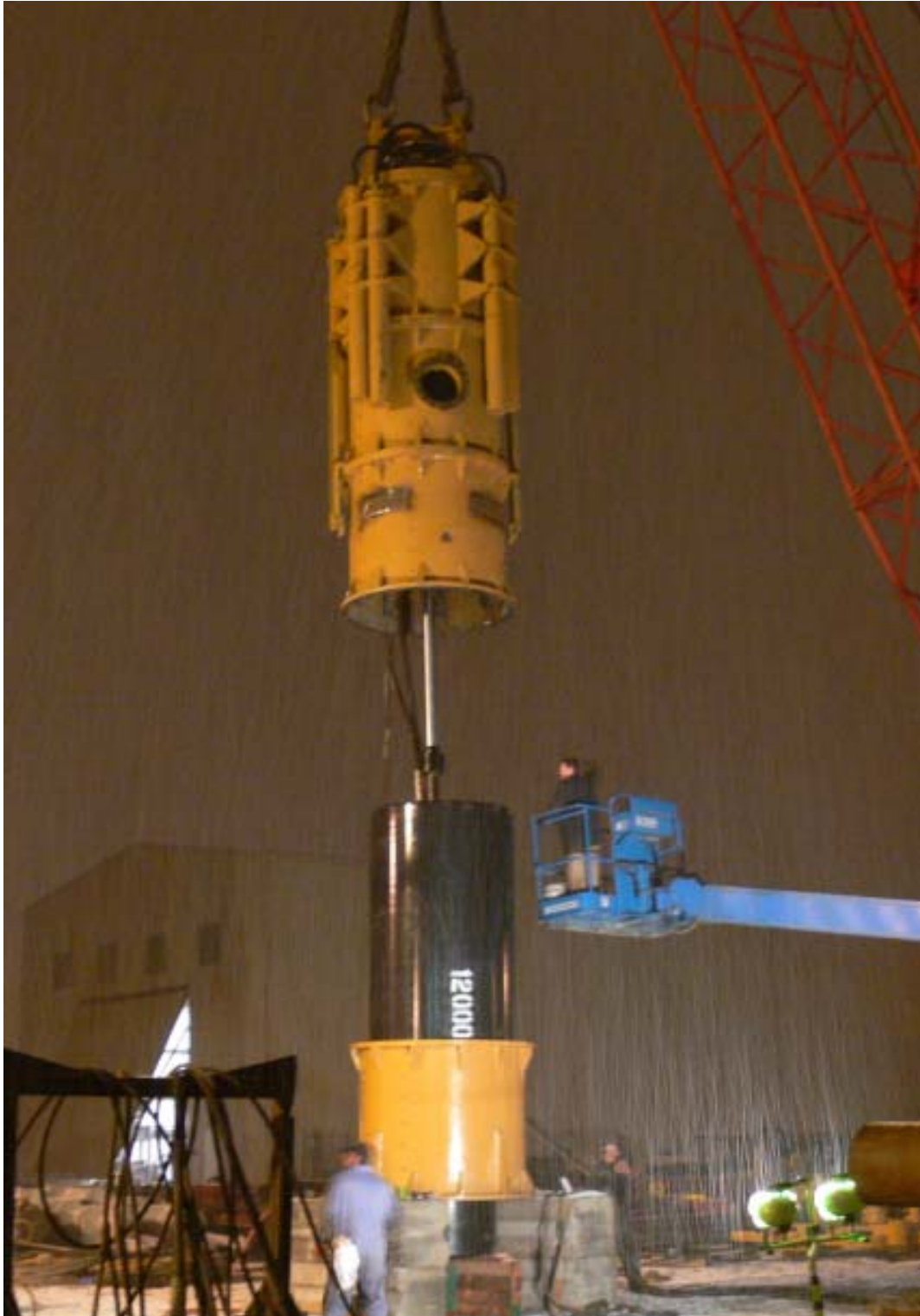
Figure 2-A. Lifting Main Cage & Cylinder onto Bottom Cage
