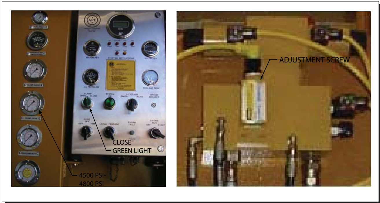
Figure 4-D. Checking Clamp Pressure Switch Setting
