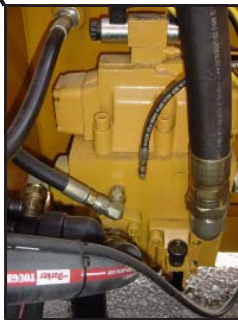
Figure 7-E. Drive Manifold Installed
