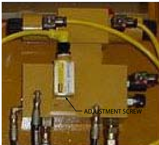
Figure 4-D. Checking Clamp Pressure Switch Setting
