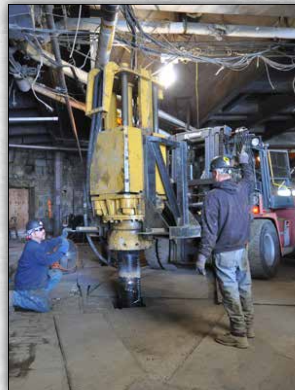
FORKLIFT MOUNTED 7.5 HYDRAULIC IMPACT HAMMER.
