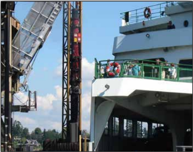
D46 DRIVING DOLPHIN PILES AT THE BAINBRIDGE ISLAND FERRY TERMINAL.
