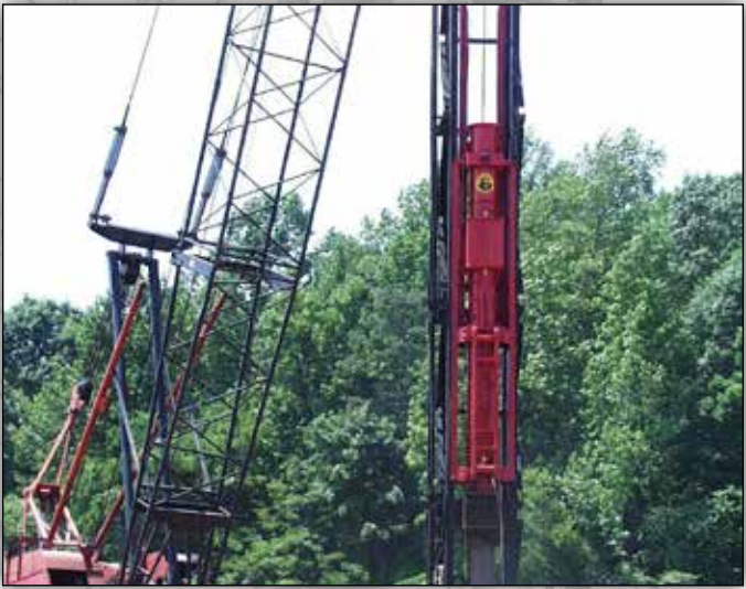
A D19-42 DRIVES H-BEAM IN NORTH CAROLINA.
