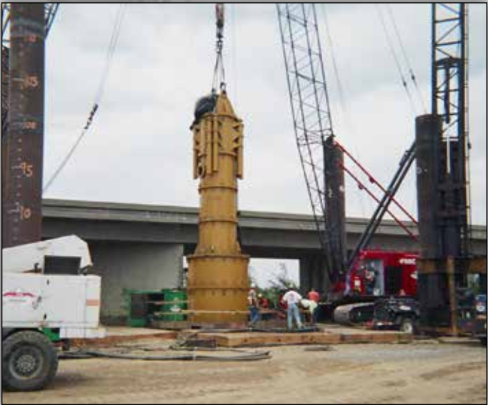
THE APE 7.5A WITH A DIRECT DRIVE BOOT.
