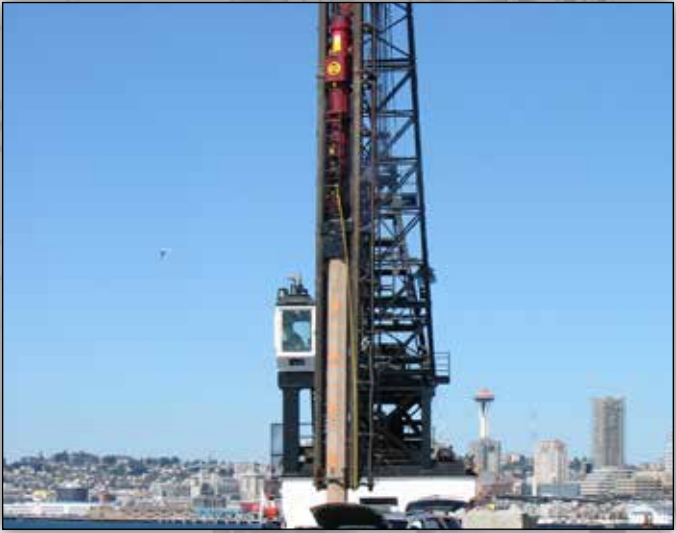
A D62 DRIVES TEST PILES AT TERMINAL 18 IN SEATTLE, WA.
