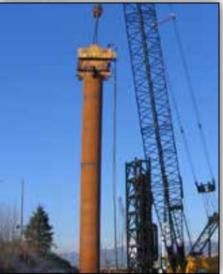
MODEL 600 VIBRO WITH THE D180-42. FINISHING 1.8 M PILES.
