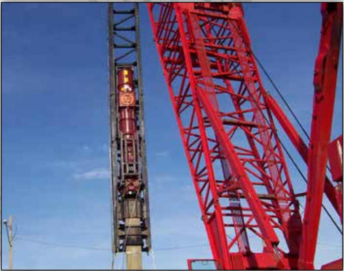
AN APE D160 DRIVES 30" SQUARE CONCRETE PILE IN OCEAN CITY, NJ.
