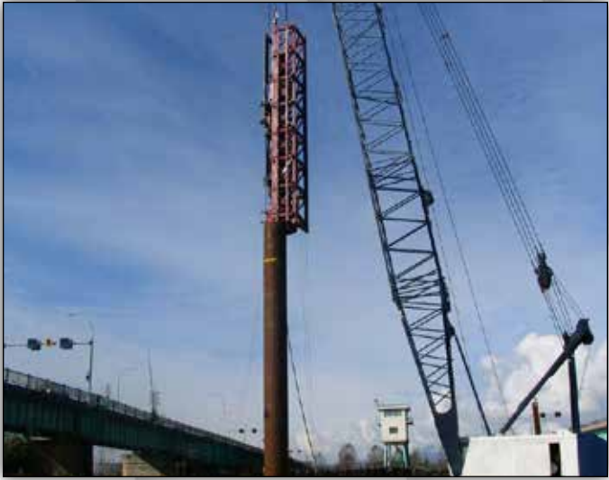
THE D180-42, LARGEST APE DIESEL HAMMER IN NORTH AMERICA DRIVES 42" PIPE PILE IN COQUITLAM, BC.
