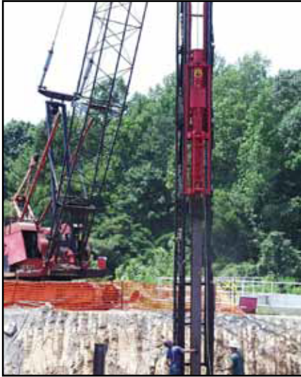
AD16-52 driving H-beam.
