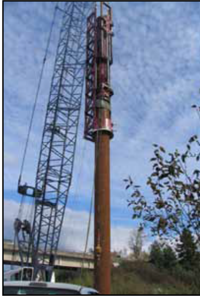
D180-42 driving 48" piles with a 54" offshore.
