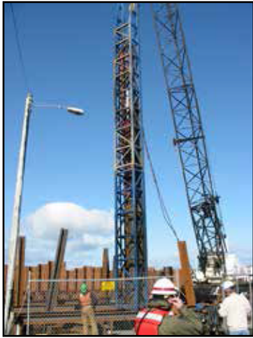
D36/26-52 Finishing Dolphin Piles.
