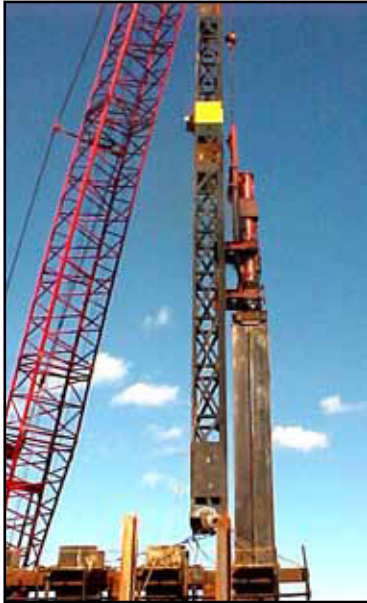
D62-52 in a stand-off driving Kingpile.
