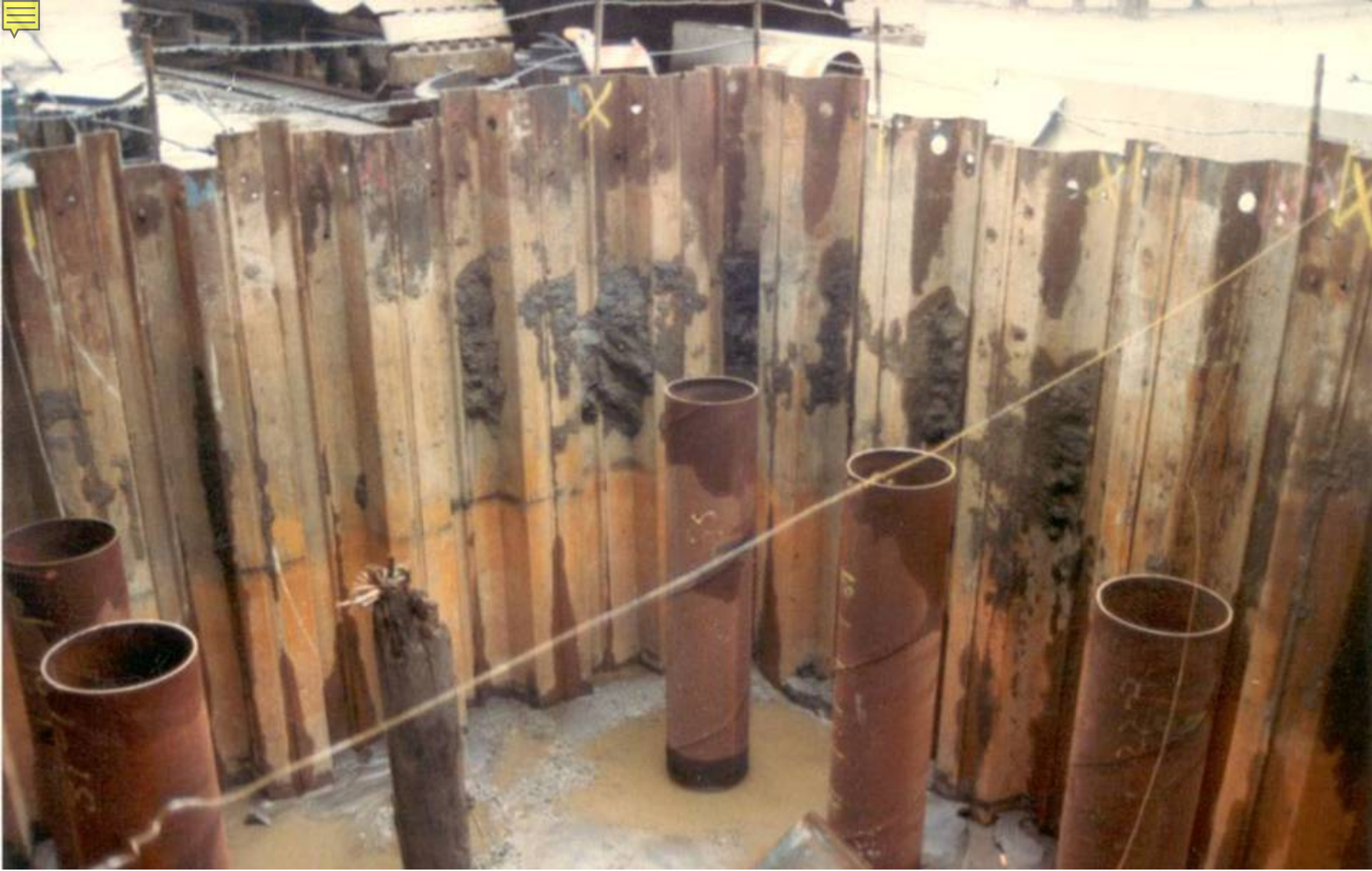
Pipe Piles inside a sheet cell
