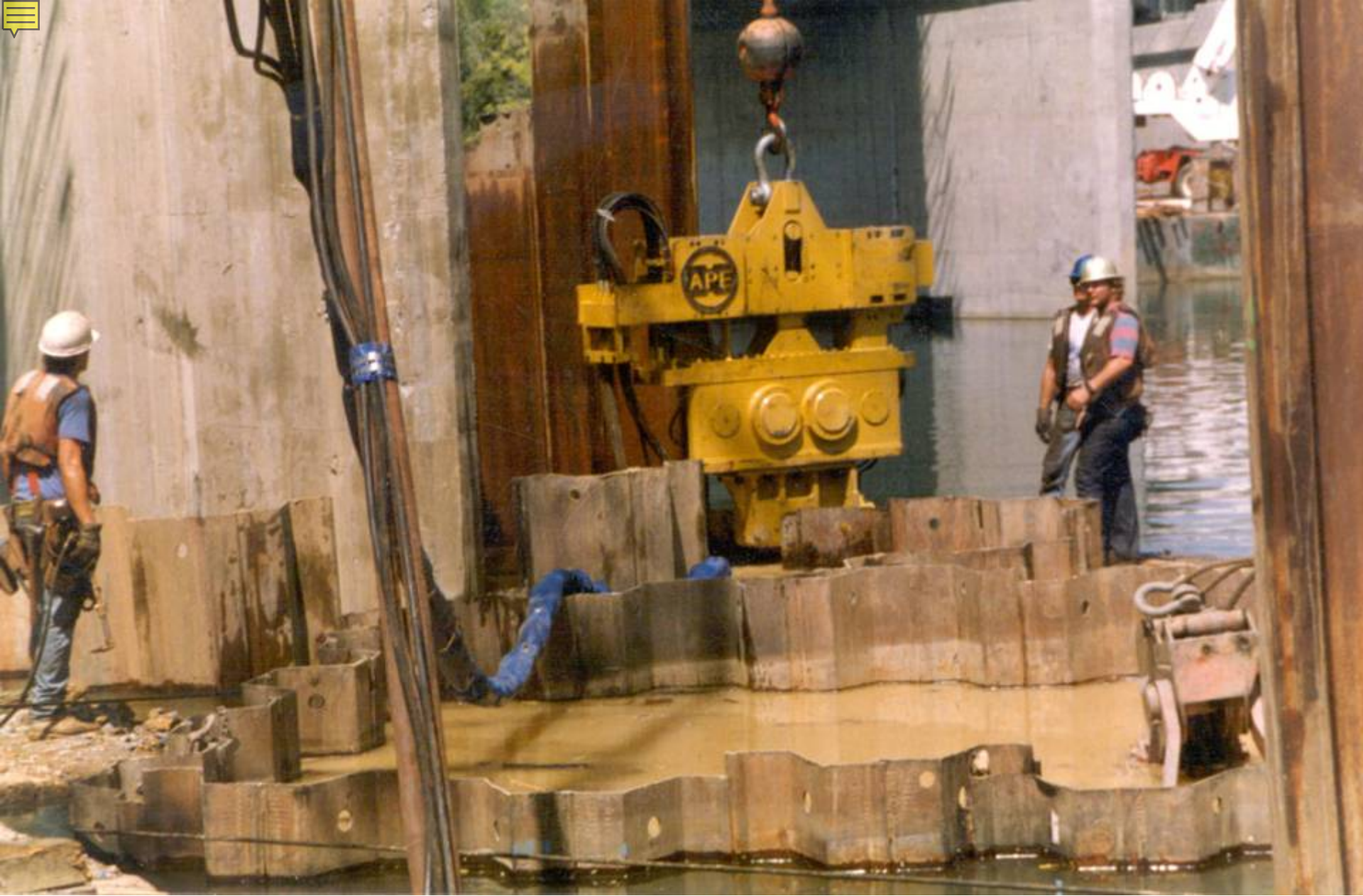
Driving a sheet pile cell in California.
