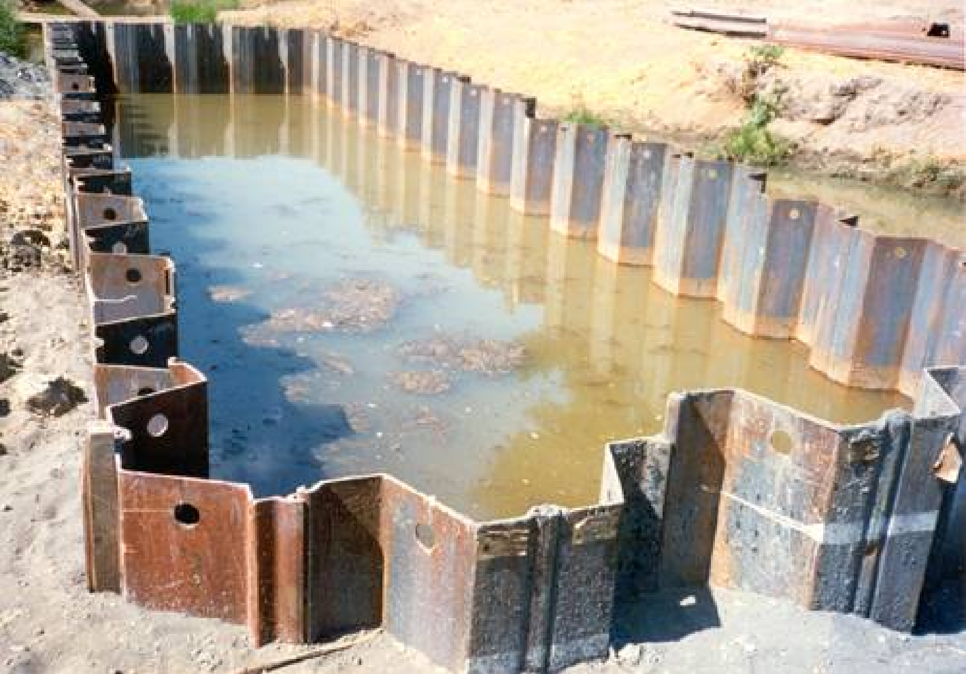
Steel Sheet Piles
