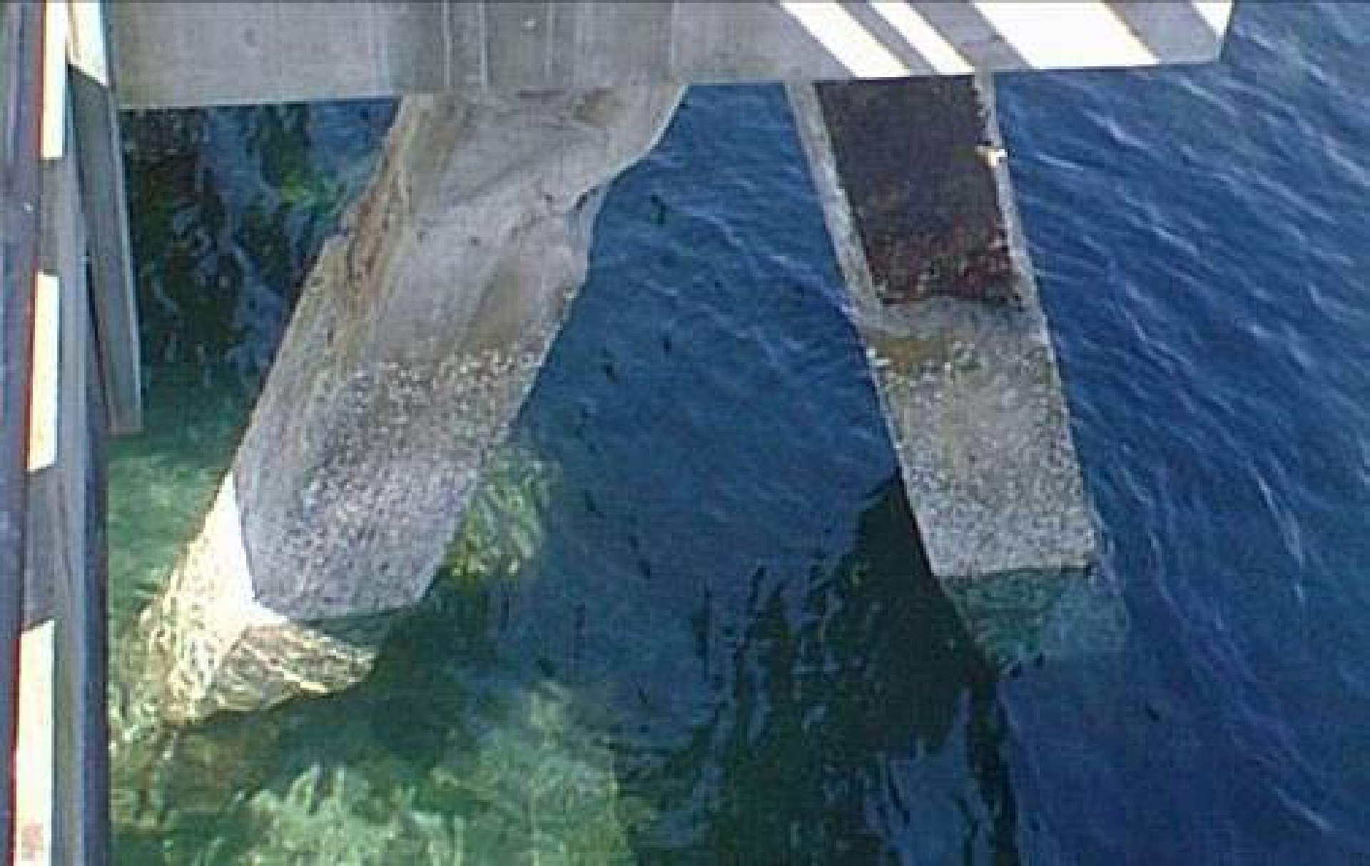
Square piles damaged by ship
