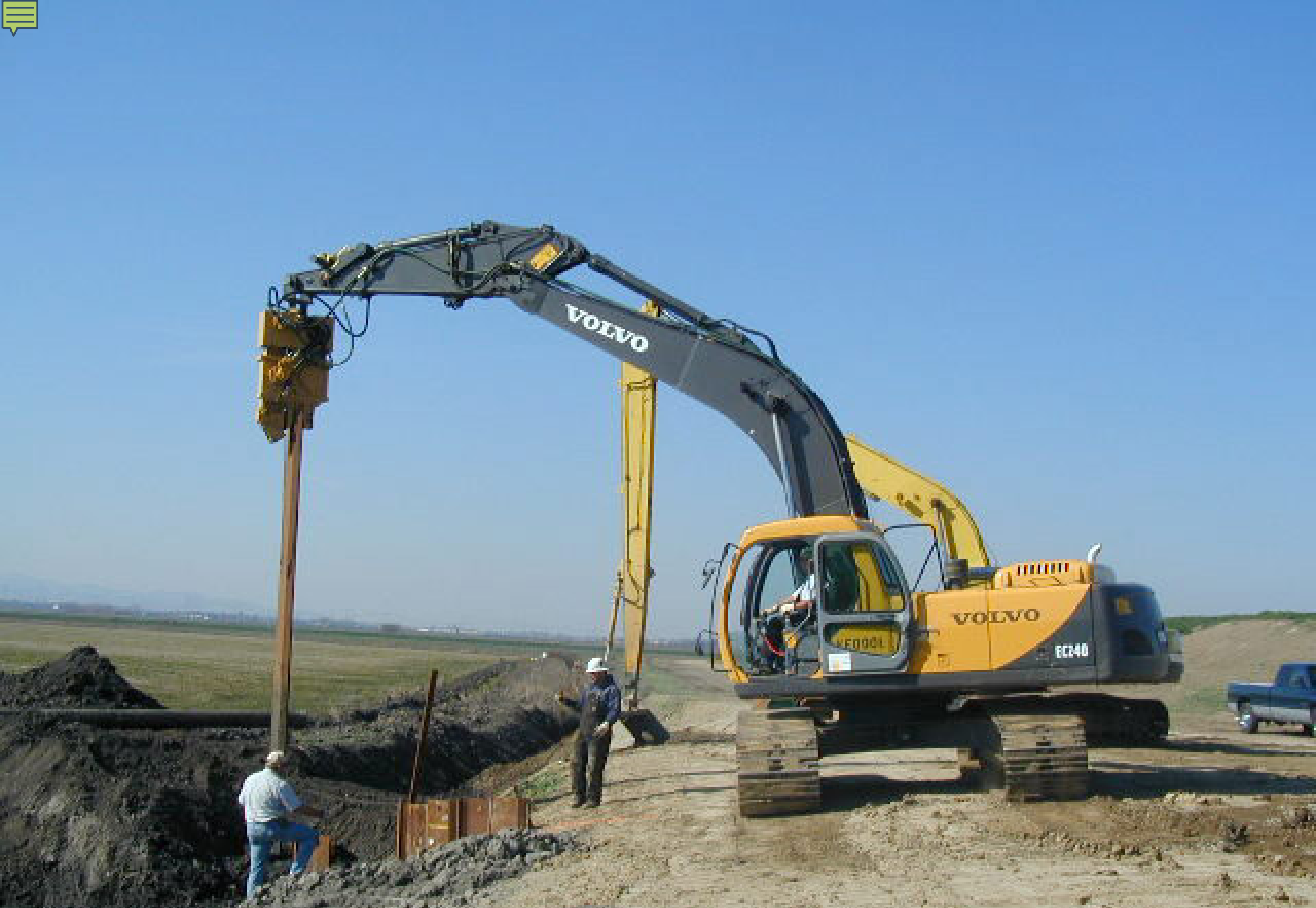
Sheets for Shoring Pipe Lines
