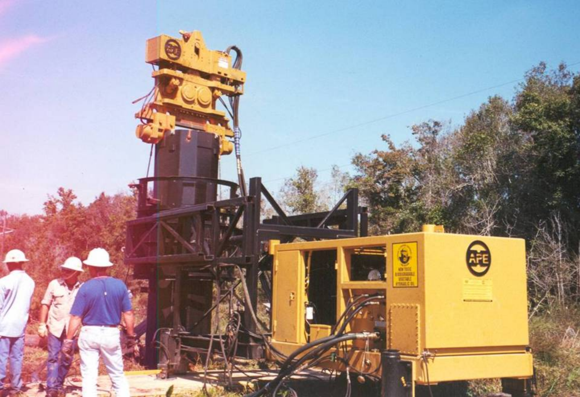
Power Pole Foundations
