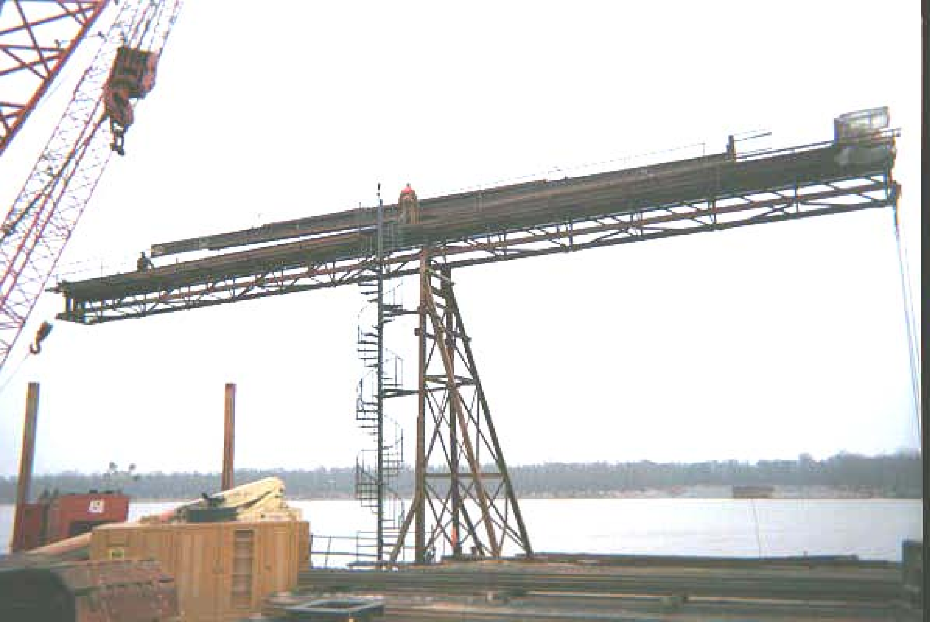
Long sheets being properly handled after extraction
