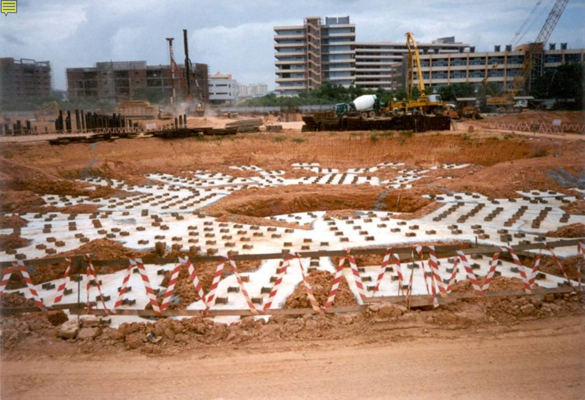
H-Beams for oil storage tanks
