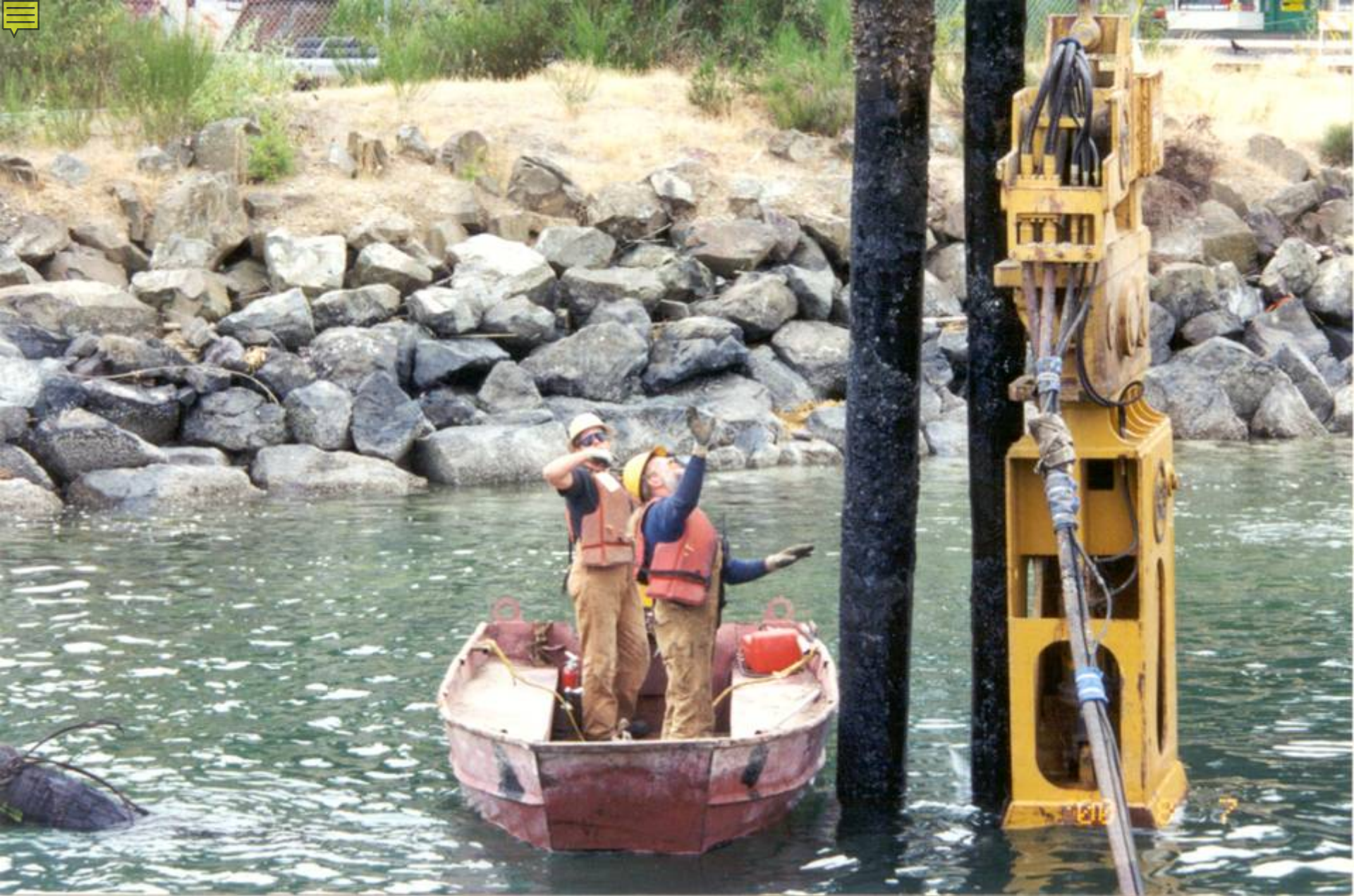
Extracting wood piles
