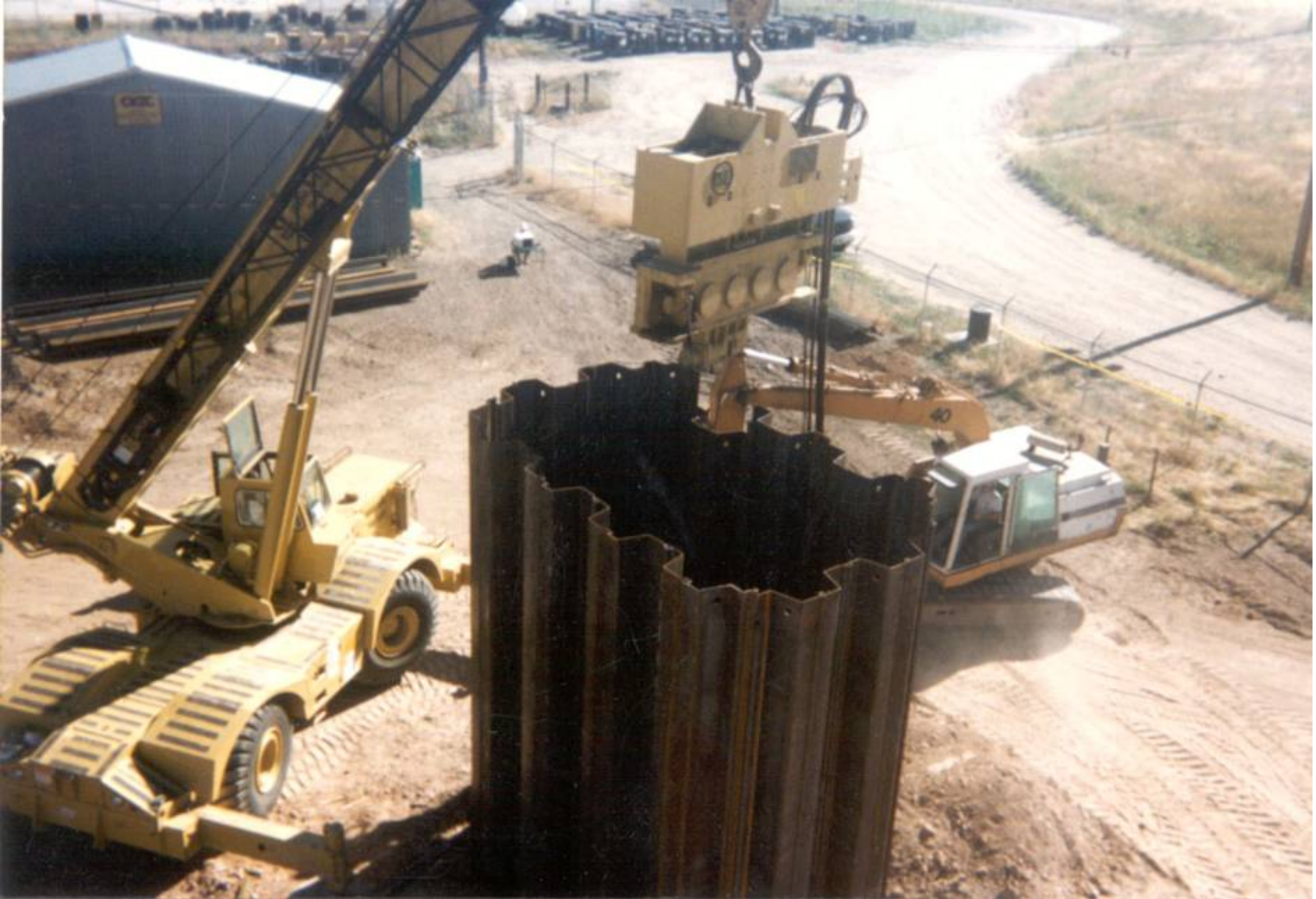
Sheet piles for Air Force missile silos
