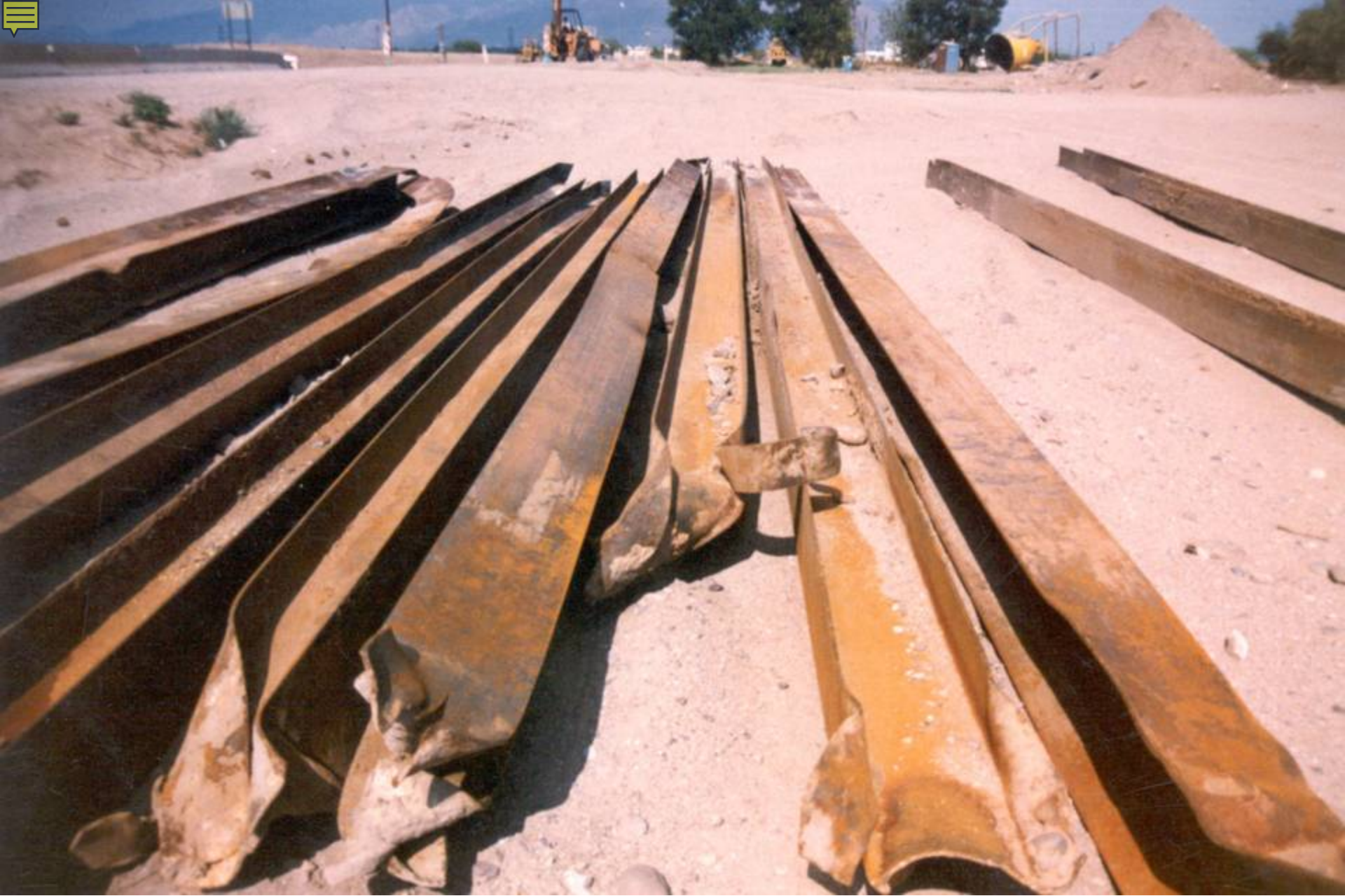
Damaged H-Beams after extraction.
