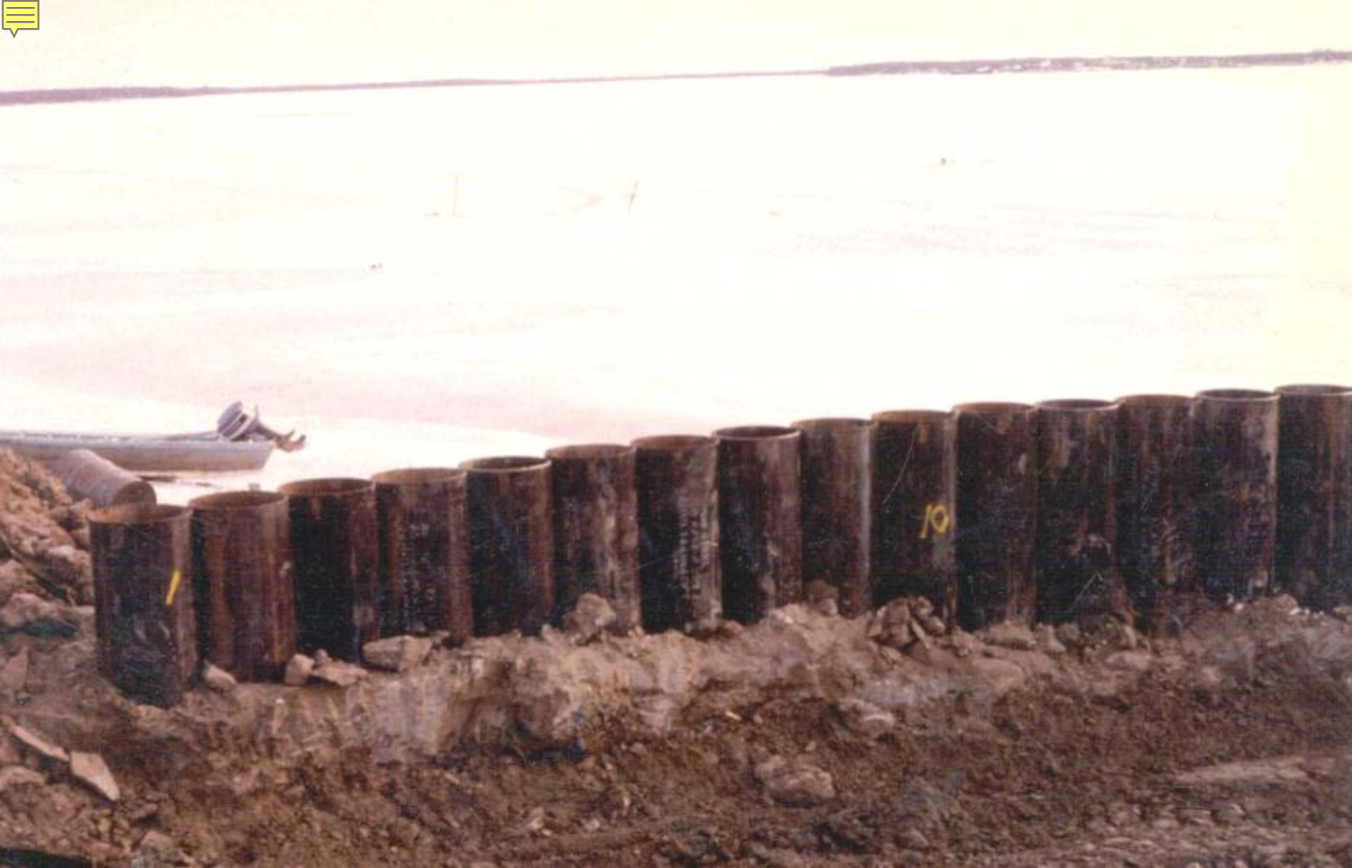
Pipe piles used to protect a river bank from ice flow damage in Bethel, Alaska
