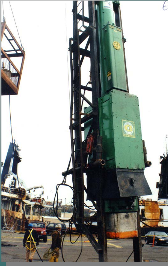
ICE 100S with sound shielding (ICE Seattle)
