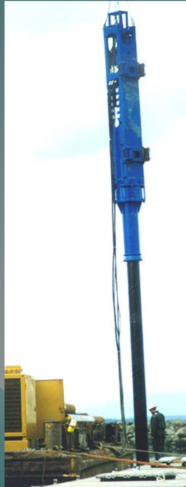
Junttan on steel pile was louder than D62
