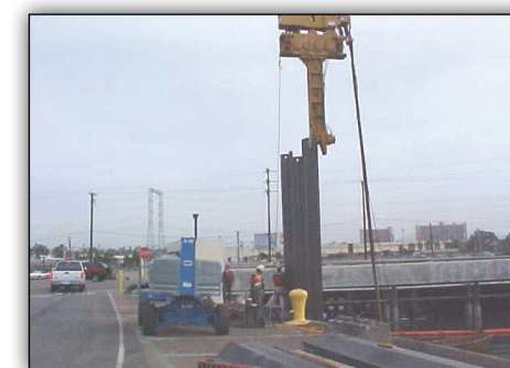
HYBRID EXTENSION CALLED THE CALIFORNIA STINGER FOR TIGHT WORKING DIMENSIONS.
